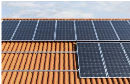
Pitched roof with tiles
