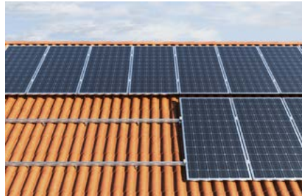
Pitched roof with tiles
