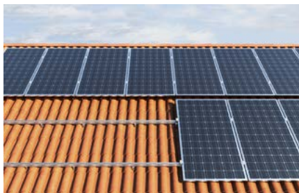
Pitched roof with tiles
