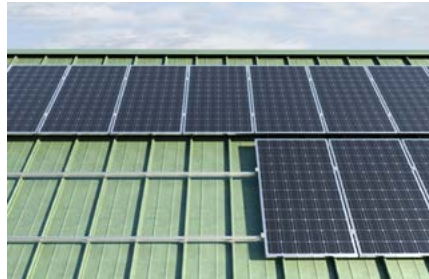
Pitched roof with rounded standing seam covering
