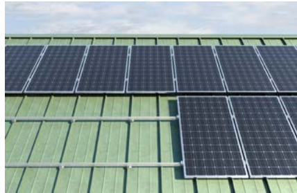
Pitched roof with standing seam covering
