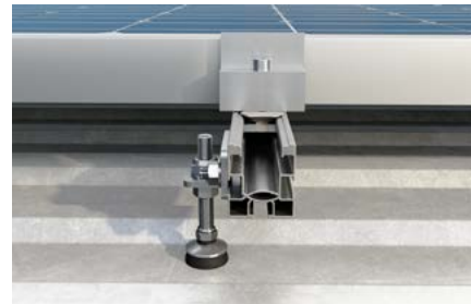
Roof with trapezoidal metal sheet covering
