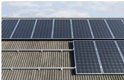
Pitched roof with corrugated sheets covering
