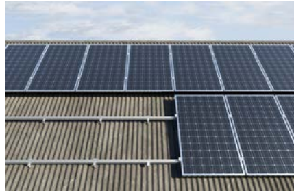
Pitched roof with corrugated sheets covering
