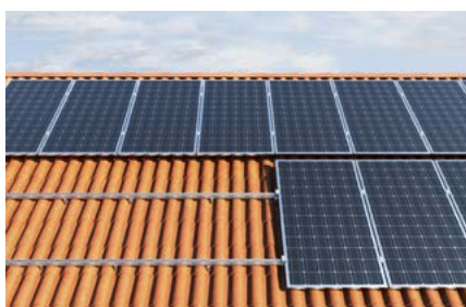
Pitched roof with tiles
