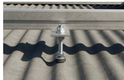
Pitched roof with corrugated sheets covering
